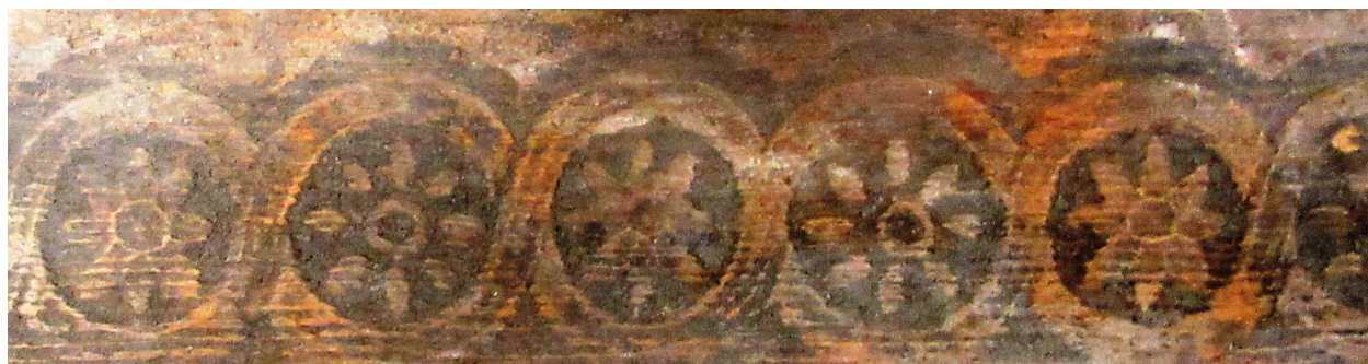
A close-up view of part of the decorative border on the Eagle Hall sign.
